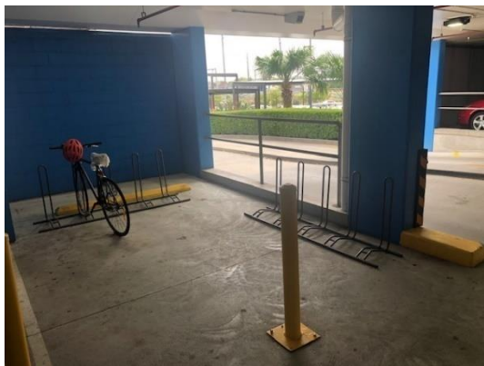
Figure 3.16: Bicycle Racks (Multi-Storey Car Park)
