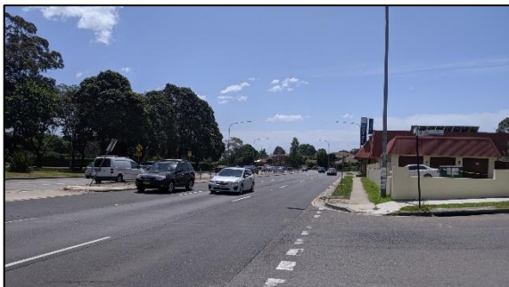
Figure 3.3: Olympic Drive (looking North)
