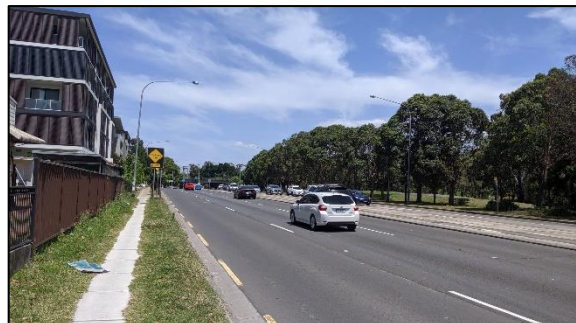
Figure 3.4: Olympic Drive (looking South)
